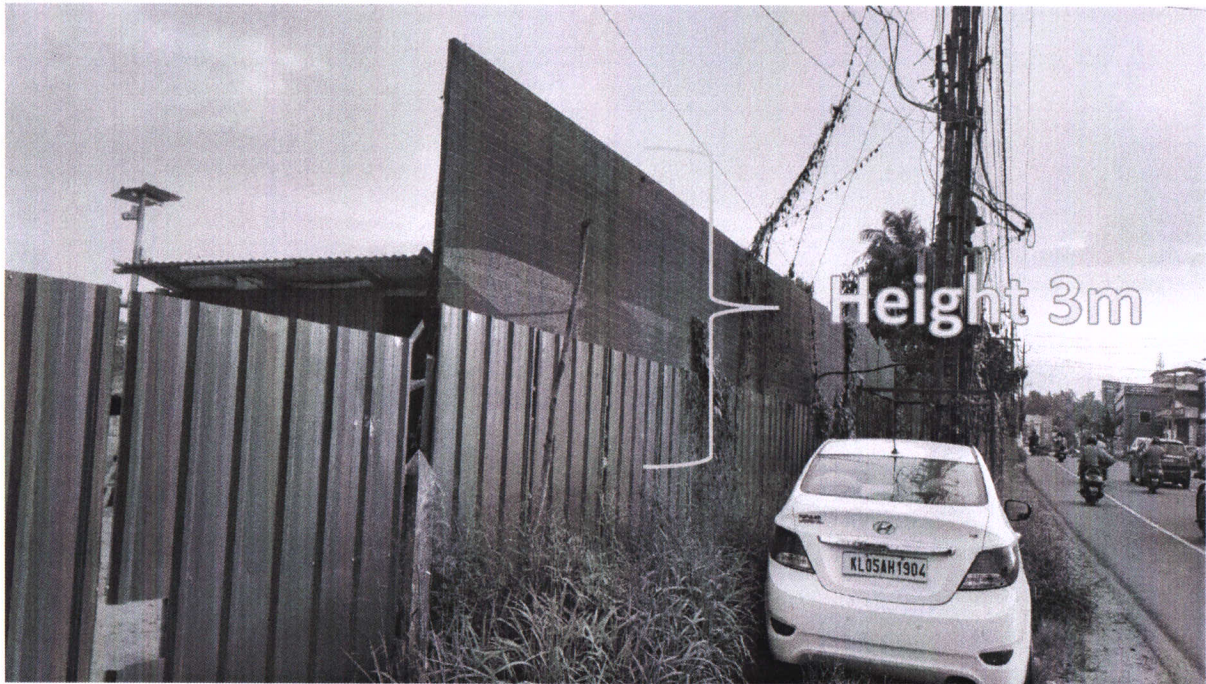
Barricading of construction site
