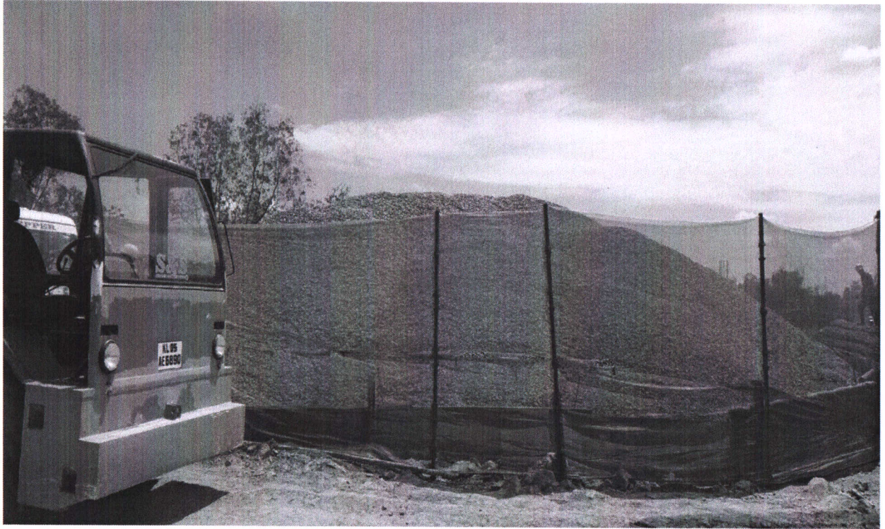
Aggregate stock at site
