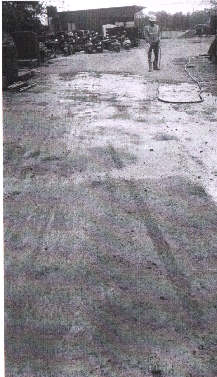
Water sprinkling over un-paved road
