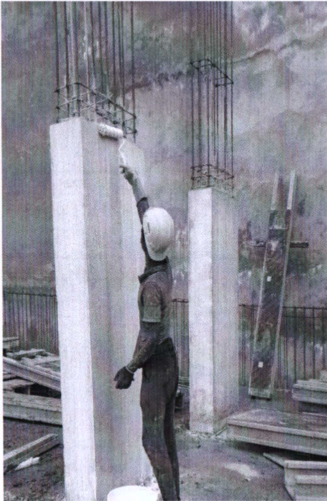
The Photograph of curing agent using at site and RMC usage
