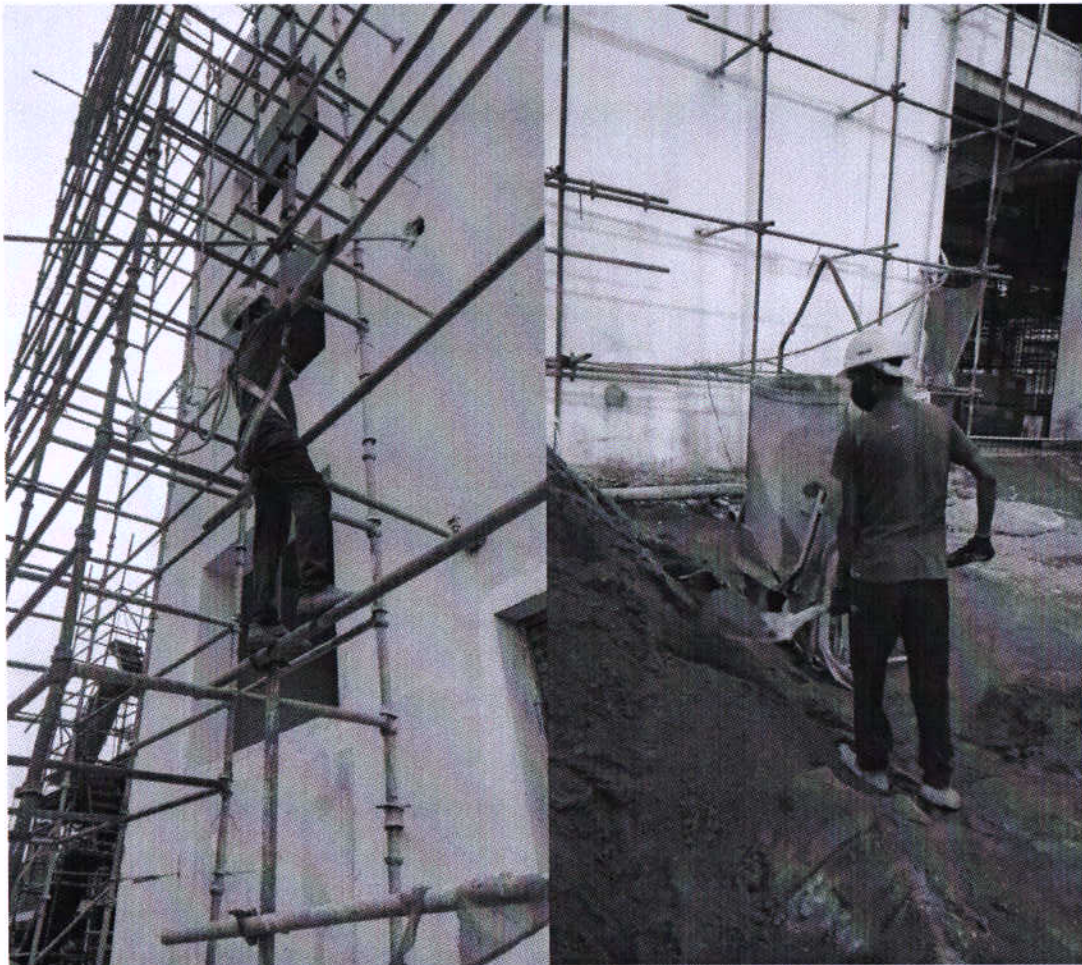
Photograph of workers using dust mask, safety harness etc.
