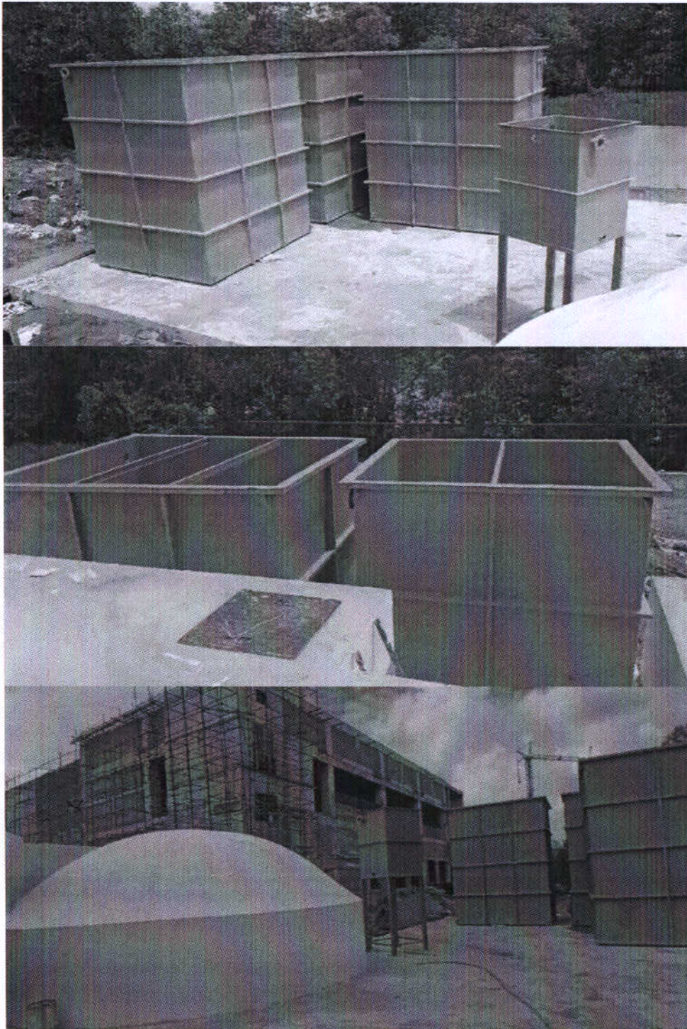
The Photographs of the STP works
